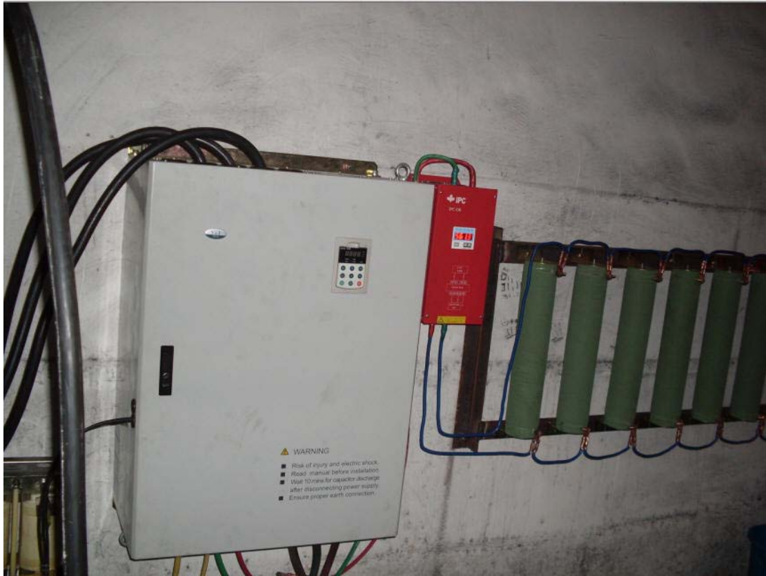
Control room of V&T EcoDriveCN variable speed drive with regenerative brake unit for mine hoist.
