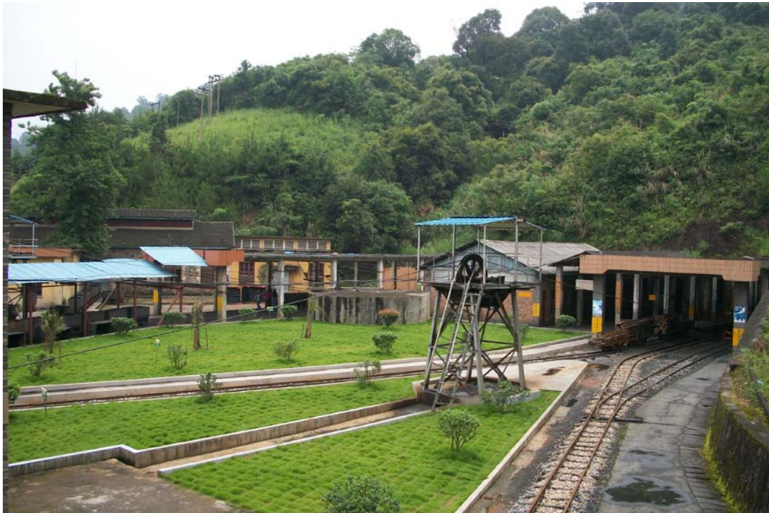
Coal winch field with EcoDriveCN drives
